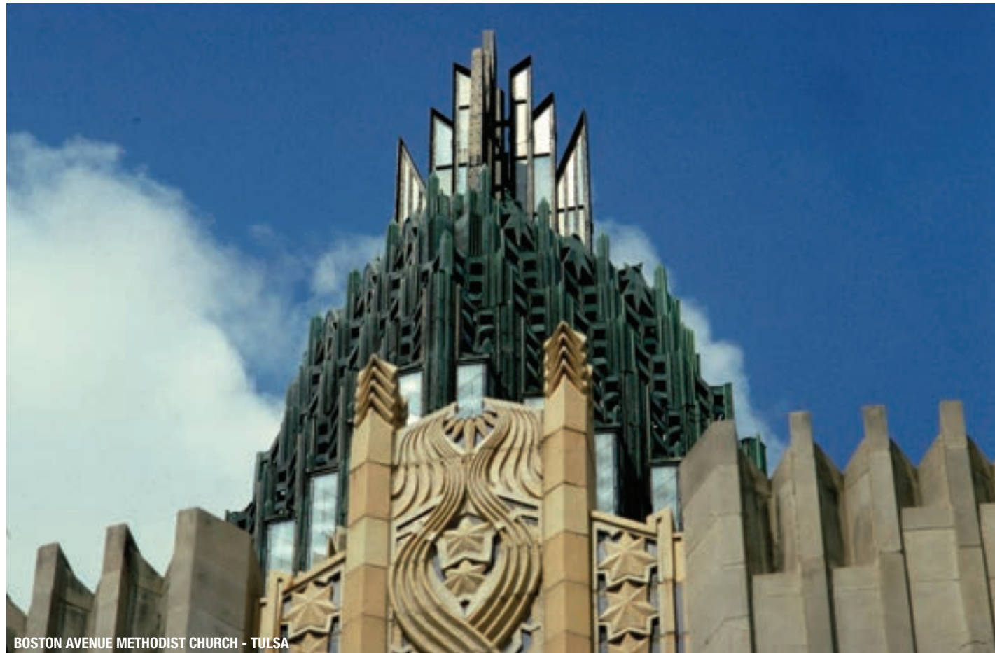
BOSTON AVENUE METHODIST CHURCH - TULSA
